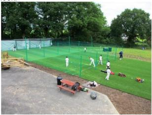
4.2 The standard size is 24m long and 2.4m high. The nets are held in place by a fixed socket system. The sockets are safely capped by a cap of artificial grass. They use a winch system to open and close the top and side nettings in a few minutes. Each lane is open ended to allow for bowlers to have a proper run-up. There is roof netting at the batter's end like so:
